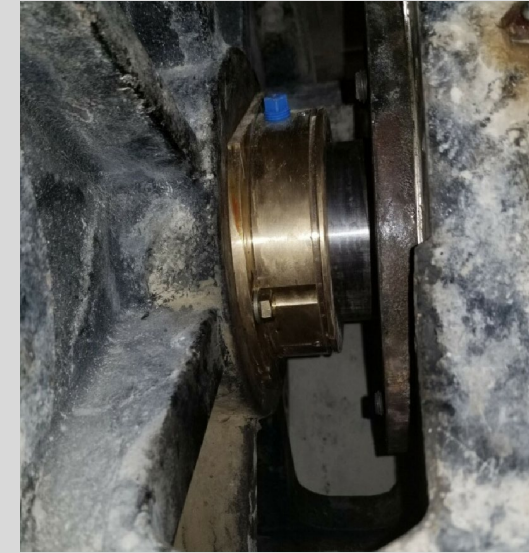
After: Air Mizer shaft seal installation
